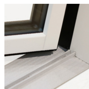
Frame IC/Nation IC low fiber threshold - terrace door
