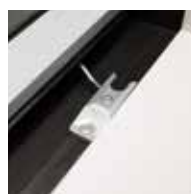
Handle operated night latch
