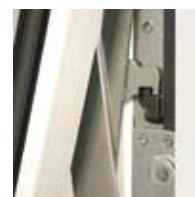
Easy clean hinges and restrictor
