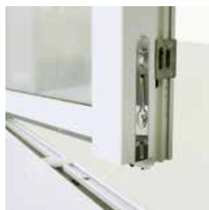
Flush bolt on floating mullion
