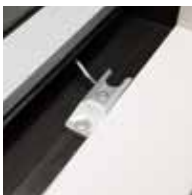
Handle operated night latch
