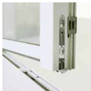
Flush bolt on floating mullion
