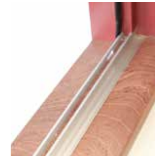
Hardwood threshold Inward opening door
