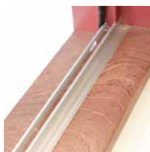
Hardwood threshold Inward opening door
