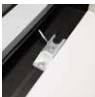
Handle operated night latch
