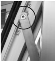
The sash, however, can be adjusted up or down slightly on the adjustment screws on the hinge.
