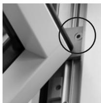
On larger opening, the frame is controlled by the built-in friction in the side mounted fitting. The friction may be adjusted by tightening or loosening the
