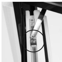
Friction brakes make it possible to hold the sash in any ventilation position, but do not provide a lock of the ventilation position.
