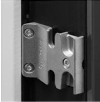
The keep has two slots, the inner slot is for closing the window, while the outer slot produces a gap at the bottom of 10-20 mm for a night ventilation facility which
