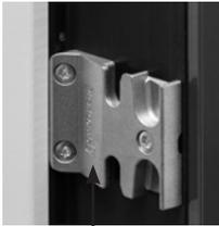
The keep is mounted with both front screws and slanted screws in the frame, which improves the window's strength against intruders.
