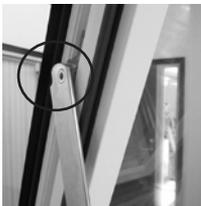
The sash, however, can be adjusted up or down slightly on the adjustment screws on the hinge.
