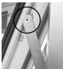
The side guided ironmongery has only very limited adjustment options, the sash can be adjusted slightly laterally by the adjustment screws on the ironmongery.
