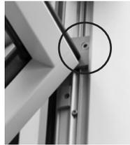
Friction can be tightened or loosened by adjusting the **friction screw** in the ironmongery on the side of the sash – to ensure easy operation and proper function, always make sure that the friction is adjusted evenly in both sides.
