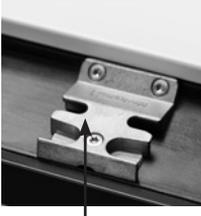
The **keep** is fitted with both front screws and slanted screws in the frame, which improves the window's strength against intruders.
