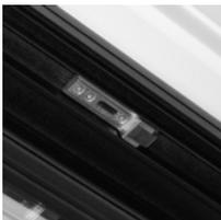
On the guide track at the top there is an end stop to ensure the door is not opened too far.
