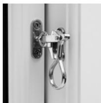
Casement catches may be adjusted by tightening or slacking the lug on the thread plate on the frame.
