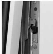
The top-swing window is equipped with an integrated child safety lock which blocks the sash when it is opened approx. 100 mm. Further
