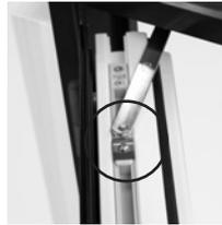
Friction brake makes it possible to hold the frame in any ventilation position, but do not provide a lock of the ventilation position. The friction
