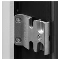
The keep has two slots, the inner slot is for closing the window, while the outer slot produces a gap of 10-20 mm for a night ventilation facility which can be securely locked in position.
