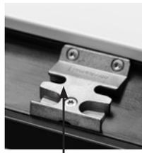
The keep is secured with both front screws and slanted screws in the frame, which improves the window's strength against intruders.
