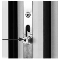
Mushroom bolts may be adjusted from time to time to increase or reduce the pressure on the sealing. The lock plate is mounted with both front screws and slanted screws in the frame, which improves strength and security.
